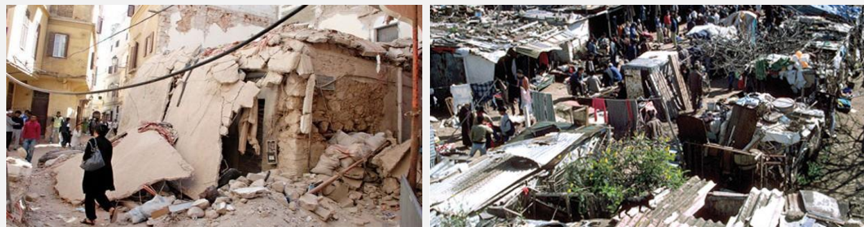
Figure 21- Homes collapsing in the Medina of Casablanca and Shantytowns in the city of Kénitra
